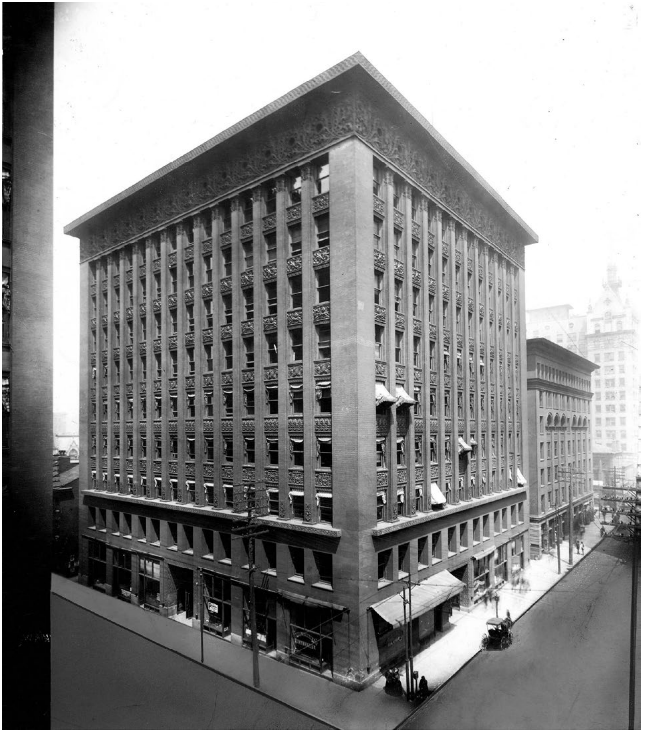
5.1.2. Louis Henry Sullivan, Wainwright Building, St. Louis, 1891, fot. Emil Boehl [Missouri History Museum Photographs and Prints Collections. Commercial Buildings. N10484]
