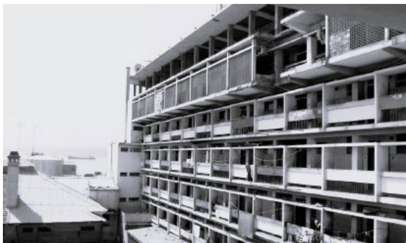
Ilustracja 2. Universal Building, Lobito, Angola (1957–1961) – Francisco Castro Rodrigues. Źródło: A. Magalhães, Modern Movement Migrations: Architecture in Angola and Mozambique (1948–1975) , „Athens Journal of Architecture” 2018, vol. 4, issue 1, s. 47.
