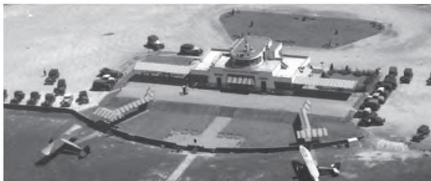
2.3-7. Washington Airport, 1930. Architekci Holden, Stott and Hutchinson.
