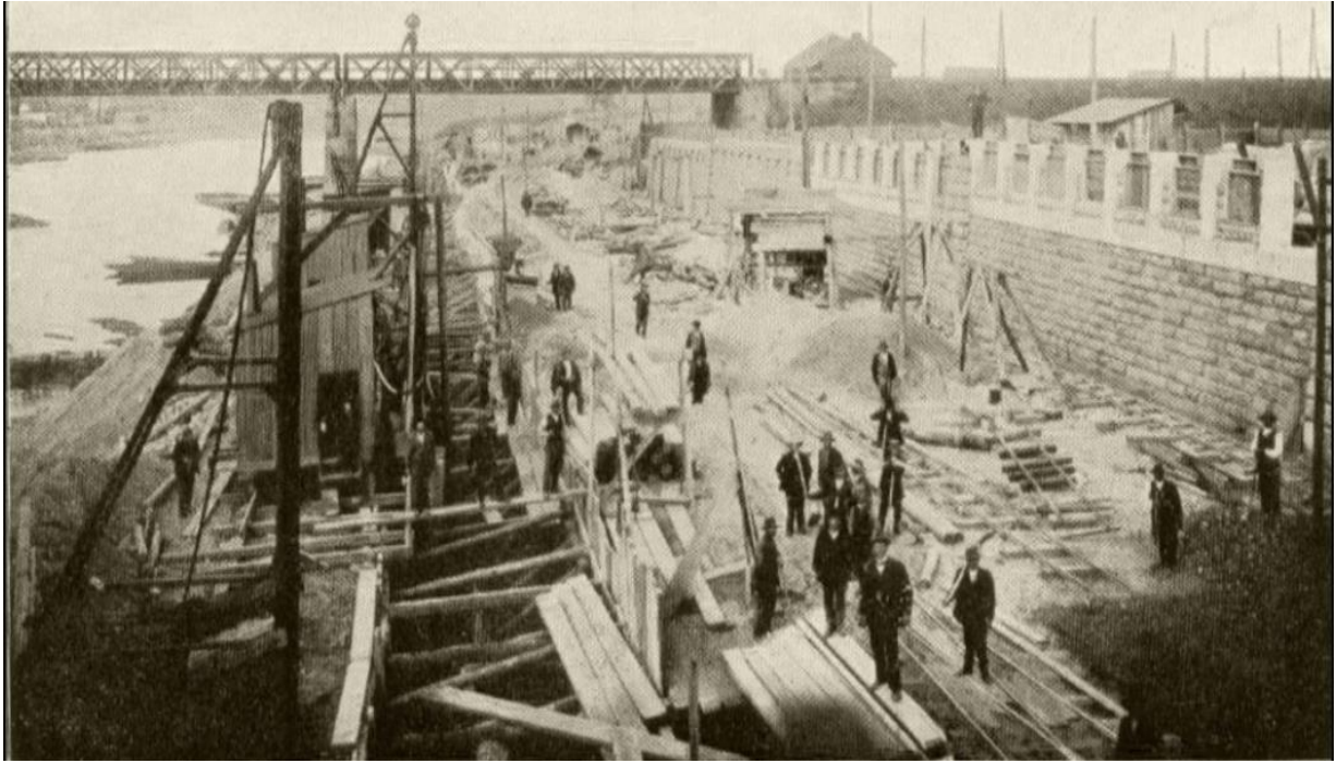
Illustration 20 – Construction of the lower right boulevard wall
