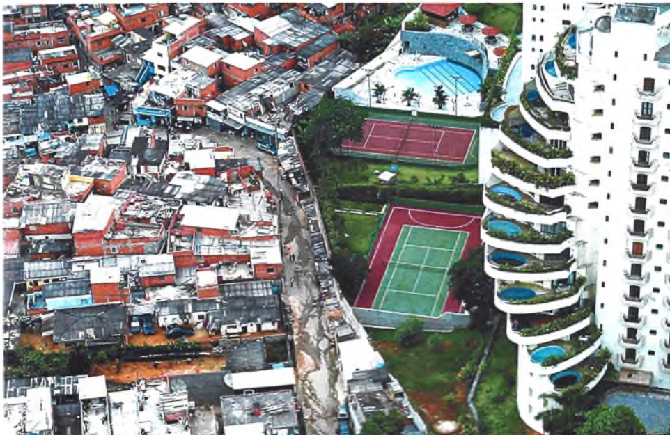
8.1 Luxurious apartments of the representatives of the upper class frequently neighbour on the slums populated by the marginalised , with only a fence separating the two; this creates a threat that “the social dynamite” will explode. Photo by Luiz Arthur Leirao Vieira.
